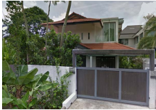
#1 PROJECT CLOSED RESIDENTIAL SOLAR PV @ Coronation Rd (10KWP)
